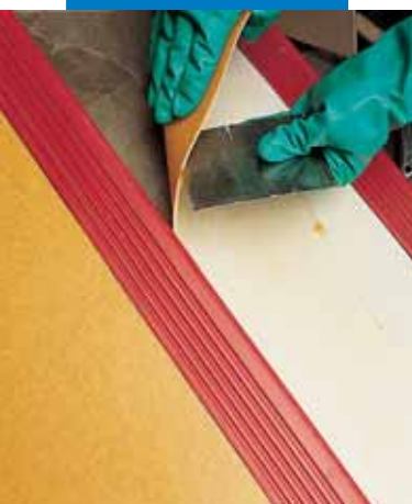
PVC installation on a step
