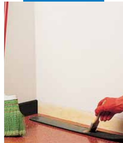
Spreading Adesilex VZ on the backing of a skirting
